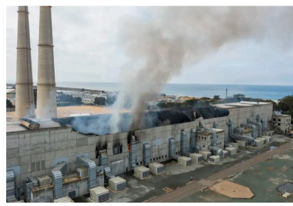
Smoke rises during a fire at Vistra Energy's Moss Landing battery storage facility in California on 17 January
