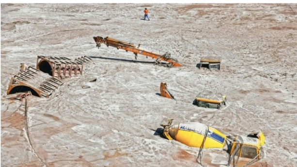
A man walks past construction vehicles covered in debris caused by flash floods after a lake burst in Rangpo, Sikkim, October 8, 2023. REUTERS
