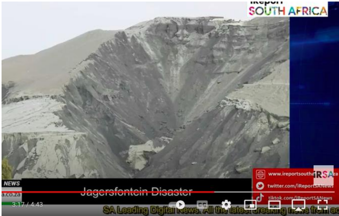
A saturated embankment can be observed
