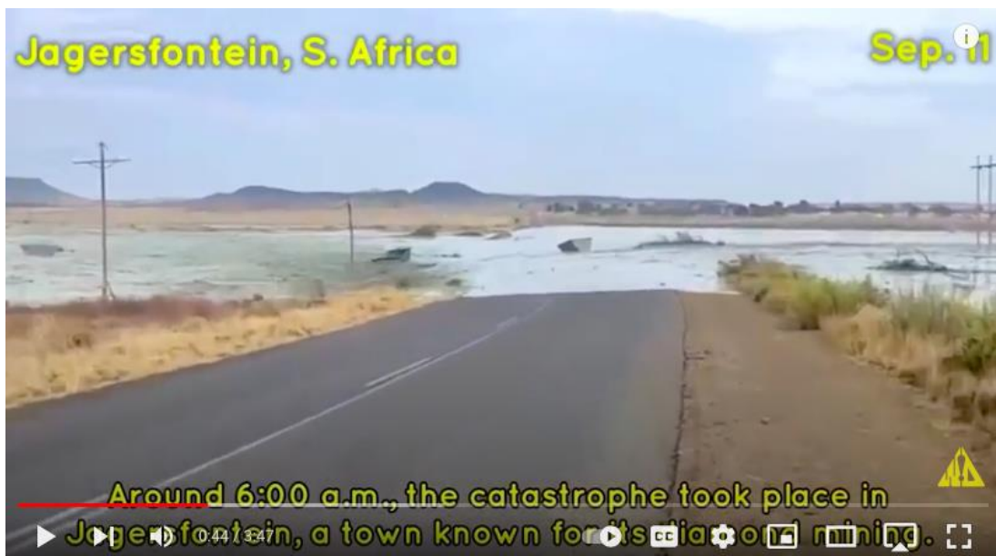
The flooding crossed an important highway
